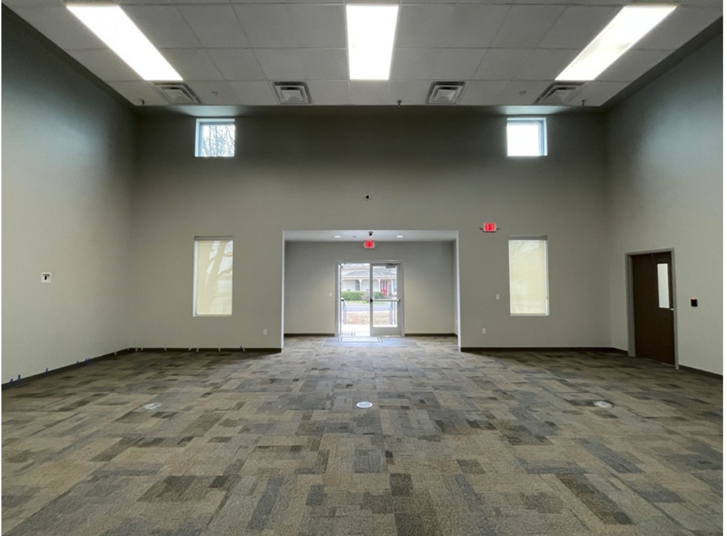
Community Center Main Room Entry View
