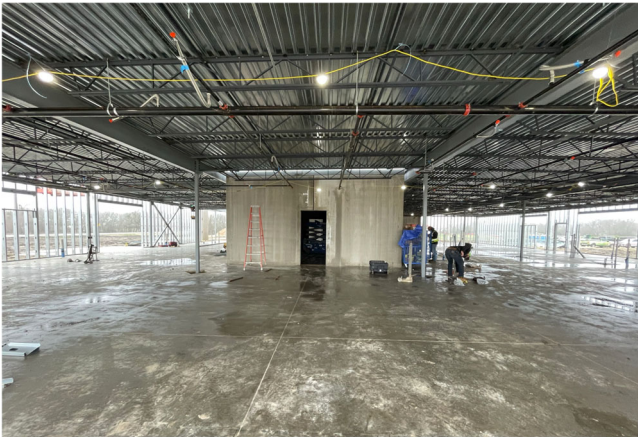
Storm Shelter View
