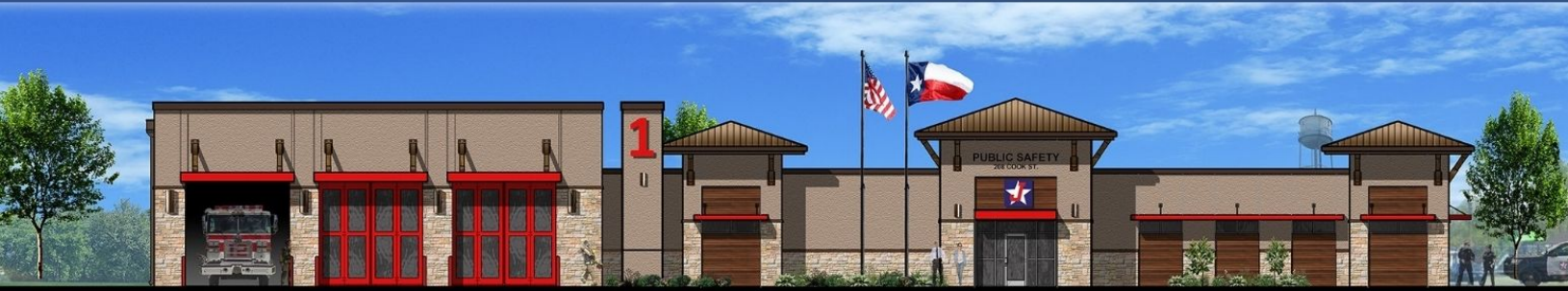
FUTURE PUBLIC SAFETY BUILDING LOCATION: 120 W. COOK ST. EXPECTED COMPLETION: FALL 2025
