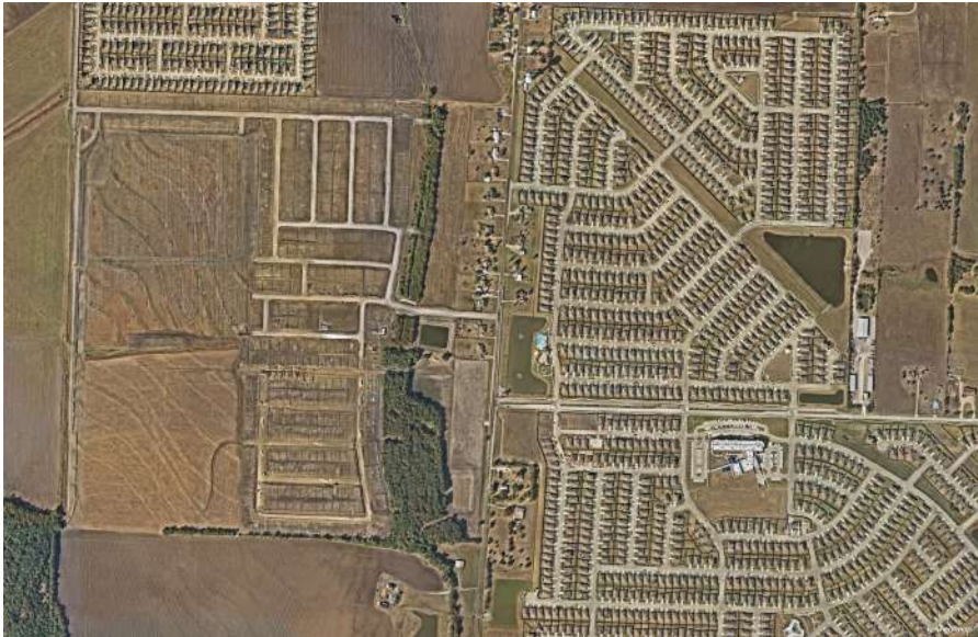
This aerial shows the Magnolia and Waverly Estates subdivisions, where the pattern of development is clear when seen from above. Source: Nearmap 2022
