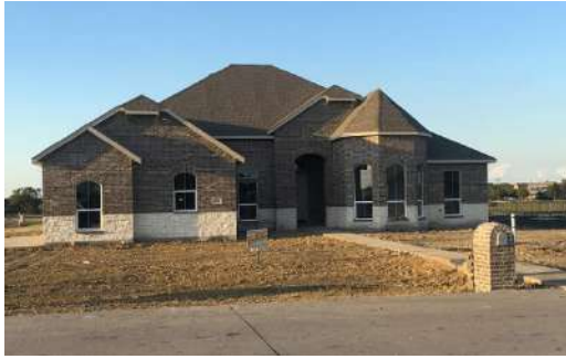
Single family home construction is driving Josephine's growth. Source: City of Josephine
