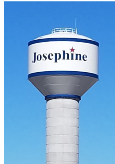
Josephine will need to continue investing in water infrastructure. Source: City of Josephine
