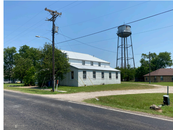
Utility poles, lines, and boxes are important factors in community appearance and should be considered in urban design standards.
